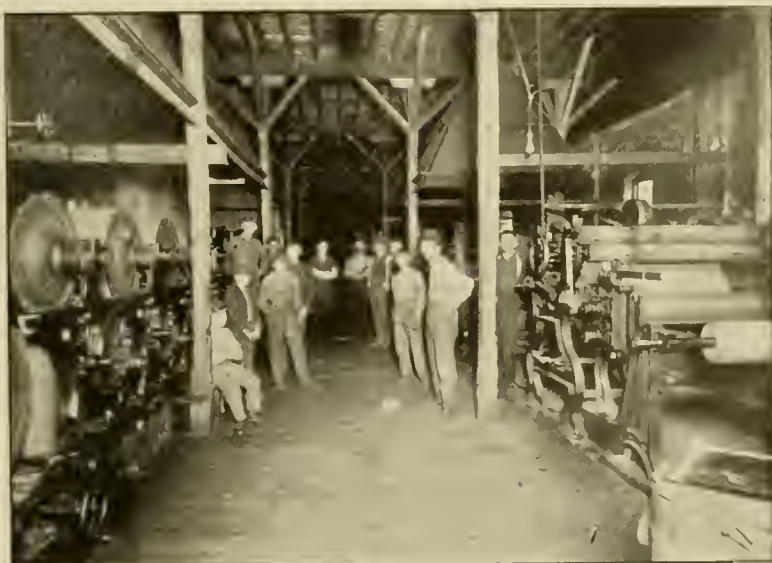
INTERIOR VIEW OF MACHINE ROOM The Ford Manufacturing Co's. Paper Mill and Roofing Plant.
